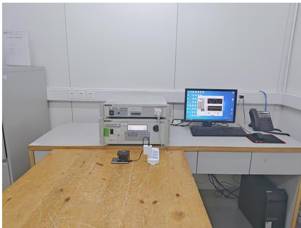
Harmonic Current Emissions & Voltage Fluctuations and Flicker
